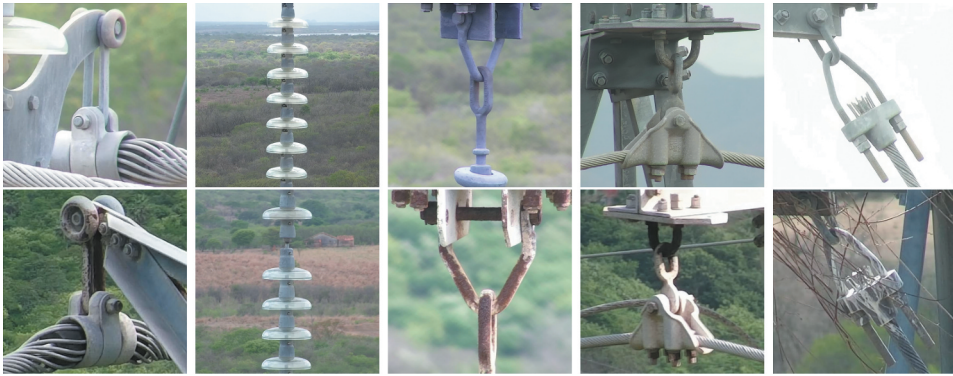
Figure 11. All five asset classes of InsPLAD-fault. The first row contains images of the assets in their normal state, and the second contains the defective assets. From left to right, the assets in the images are Yoke Suspension (normal/rusty), Glass Insulator (normal/missing cap), Polymer Insulator Upper Shackle (normal/rusty), Lightning Rod Suspension (normal/rusty), and Vari-grip (normal/bird's nest). Vari-grip can also be rusty.
