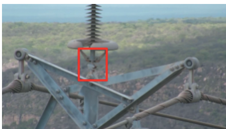
Figure 5. Polymer Insulator Lower Shackle.
